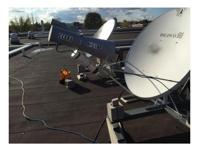
The dishes are mounted using the manufacturer-supplied mount, with additional reinforcement. The mount is then attached to a "footing" consisting of crossed  $2 \ge 6$ " lumber, with concrete half-blocks to provide adequate hold-down mass.
